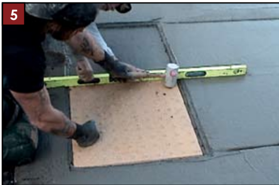
5 Set CASTinTACT® with rubber mallet. Wedge or flared edge of panel facing the curb. Check slope with level.
