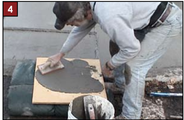
4 Pre-dampen and parge the back of the panel with CASTinTACT® Premix or fresh concrete.
