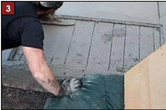
3 Remove the INSTALaTACT® tool and level concrete base with wood float.
