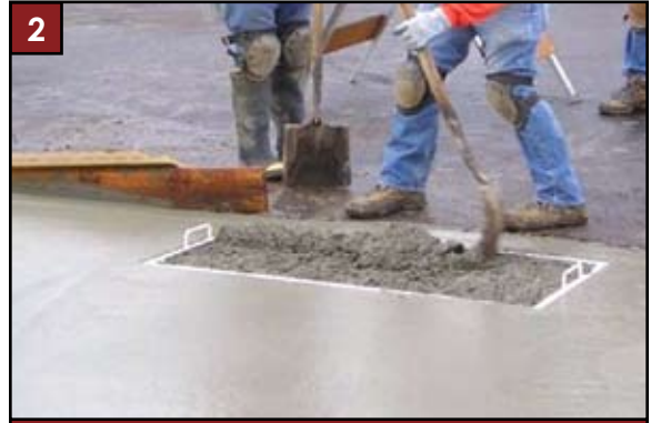
2 Removal of concrete is fast & easy with a square point shovel.
