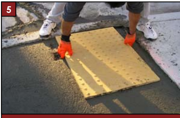
5 Place CASTinTACT® into fresh concrete 6-8" from curb line and set panels with a rubber mallet. Wedge or flared edge of panel facing the curb. 2" minimum new concrete all sides.
