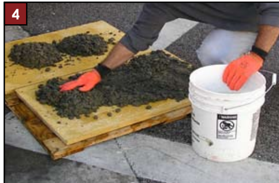
4 Pre-dampen and parge back of panel with CASTinTACT® Wet Set PreMix or fresh concrete.
