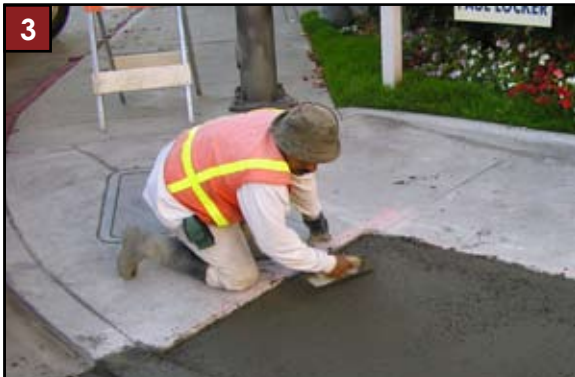
3 Concrete shall be poured, leveled, floated and recessed 7/8" below finish grade.
