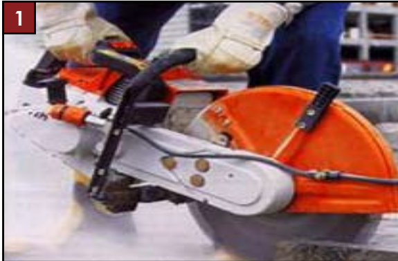
1 Predetermine measurements prior to cutting, oversize all sides minimum 2" each direction.
