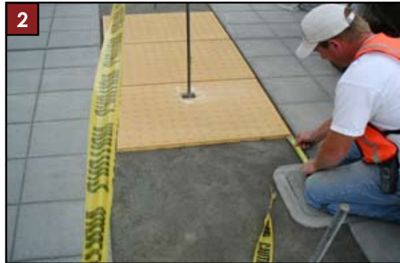
2 Measure tactile area for precutting of panels.
