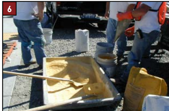
6 Pre-Mix grout and color pigment to match CASTinTACT® panels.
