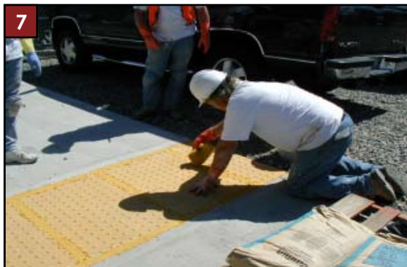
7 Expansion and panel joints must be installed and in compliance with TCA EJ171.
