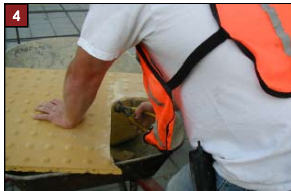
4 Panels can be radius cut around vault boxes.
