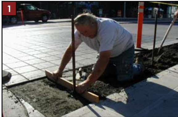
1 Finish substrate 1-3/8" below finish grade.
