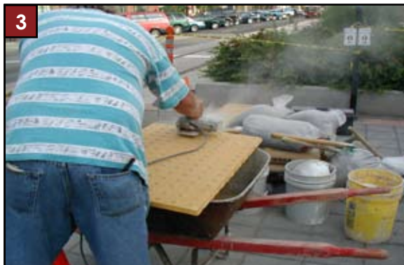
3 Panels can be easily cut with diamond blade.
