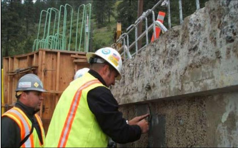
Perry Arch Bridge Beam repair using Tamms Speedcrete PM first Test Patch.
