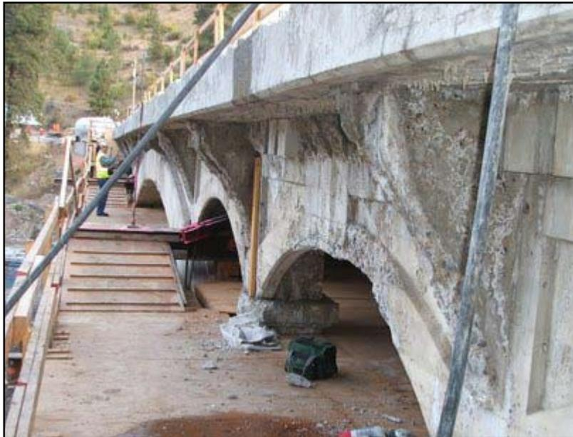
Perry Arch Bridge false work. Preparing arches for concrete repair using Tamms Form & Pour Material.
