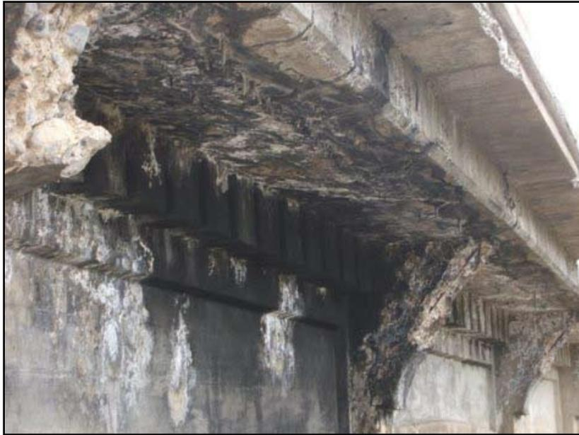
Perry Arch Bridge Corbels to be removed and replaced.
