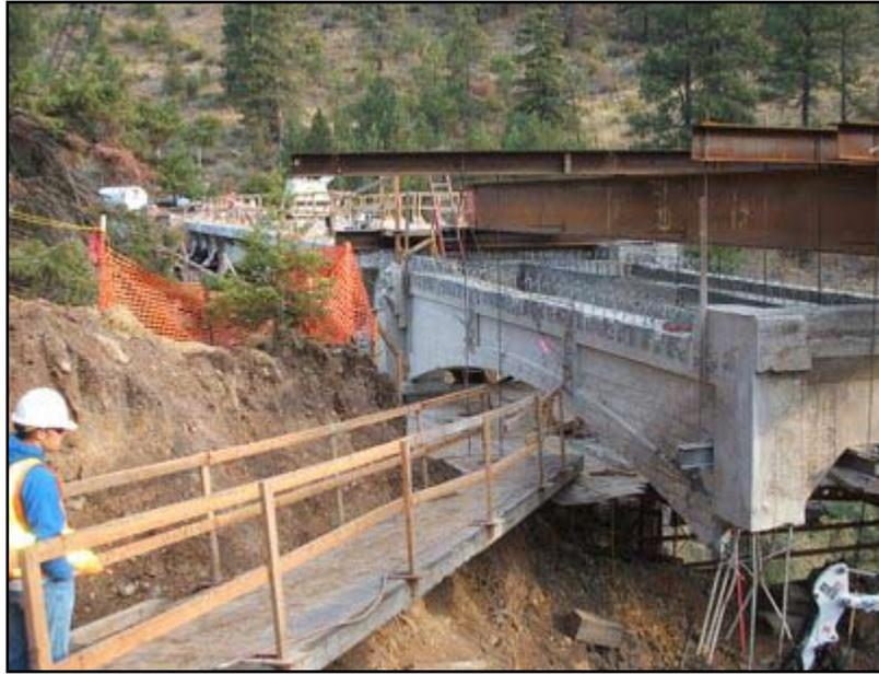
Perry Arch Bridge South end suspended off temporary I-Beam in order to replace footings.
