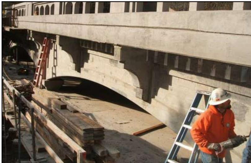
North end final repair on corbels and arch beams.
