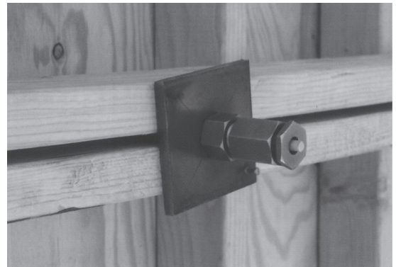
Rod, Gripper and Bearing Plate - the basic components of the Light and Medium Systems
