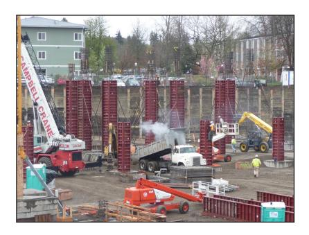
24" x 24", 24" x 42", 30" x 30", 36" x 36", and 36" x 48" square and rectangular columns 26'-0" high to support arena concourse level. Formed with All Steel "ACF" Adjustable Column Form System with welded steel chamfer.
